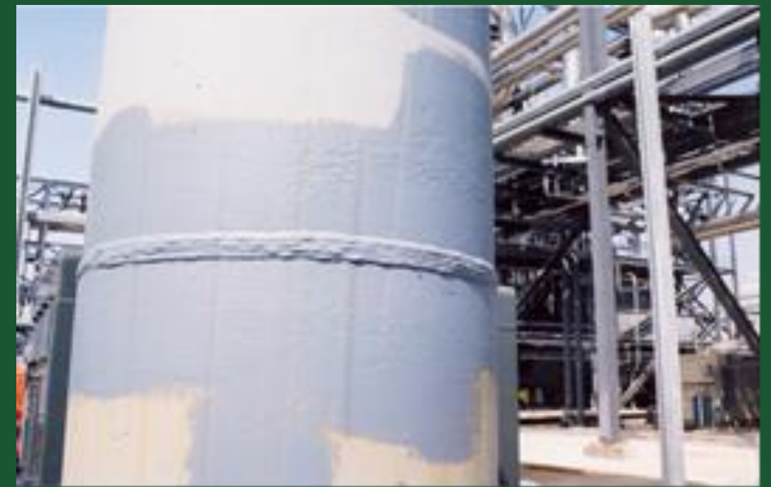
Figure 2: Weld joints were spot primed with Si-COAT 579 for added protection
