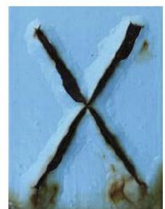
Two-coat IOZ/ polysiloxane-epoxy copolymer system applied to steel abrasive blasted to white metal
