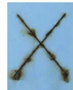
Three-coat IOZ/epoxy/PU system applied to steel abrasive blasted to white metal
