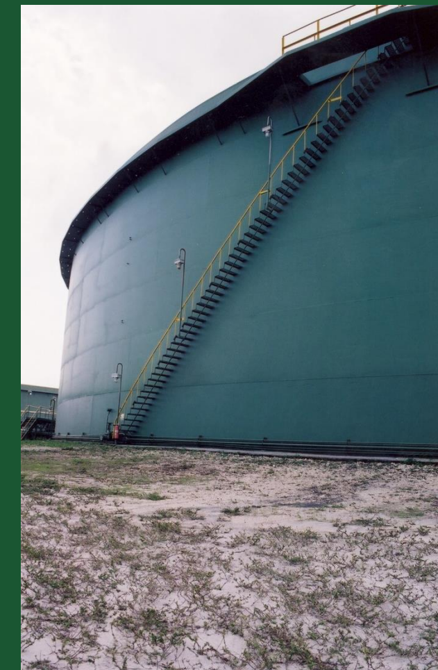
Primerless, one-coat Si-COAT 579 AC system applied directly to rusted steel.
